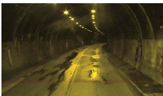
g) M17, Tunnel Crnaja km 15+082
