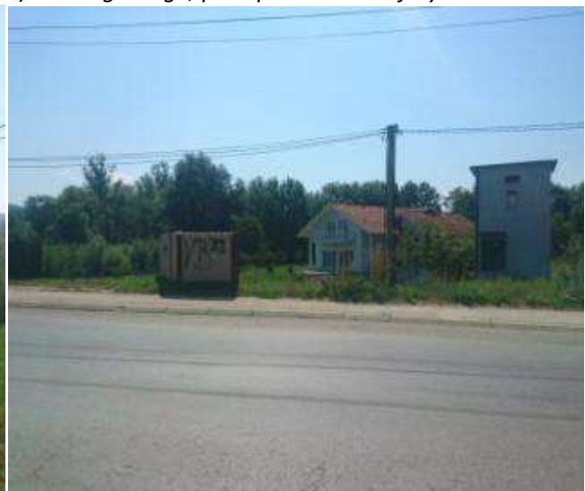
f) future connection point of the temporary bypass and the existing main road
