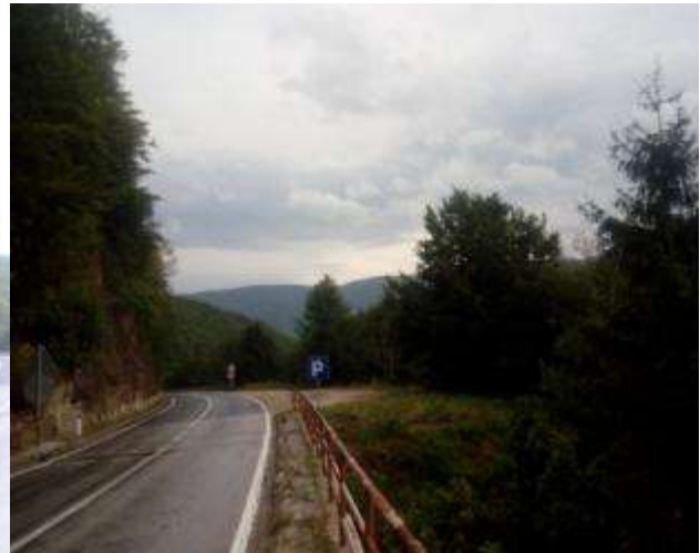
d) existing bridge
