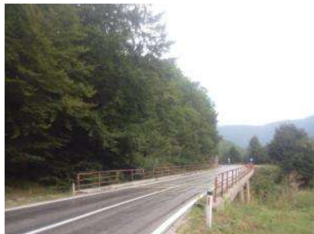
b) existing bridge
