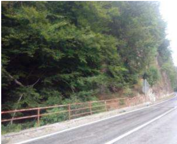
c) existing bridge
