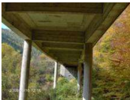
a) Span structure
