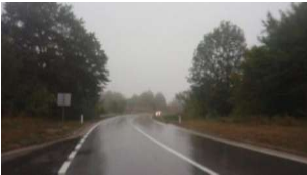
a) land alongside the project section
