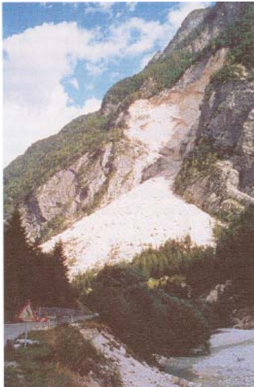
Figure 6.38: Extensive rock fall in Trenta - the major road can be protected only by a gallery
