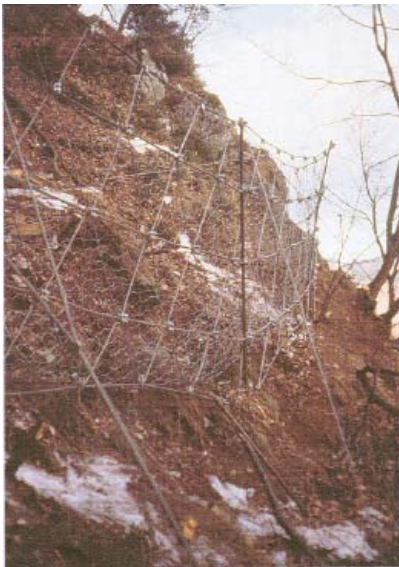
Slika 6.46: Snow nets above Hrušica Vrba motorway offer protection against rock falls and snow avalanches
