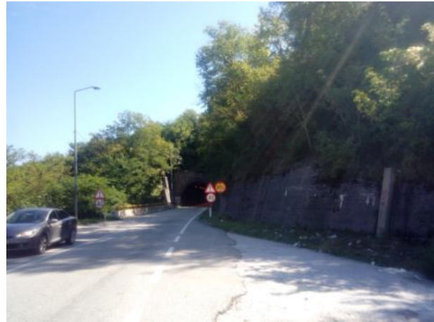
b) public land at the west exit of the tunnel
