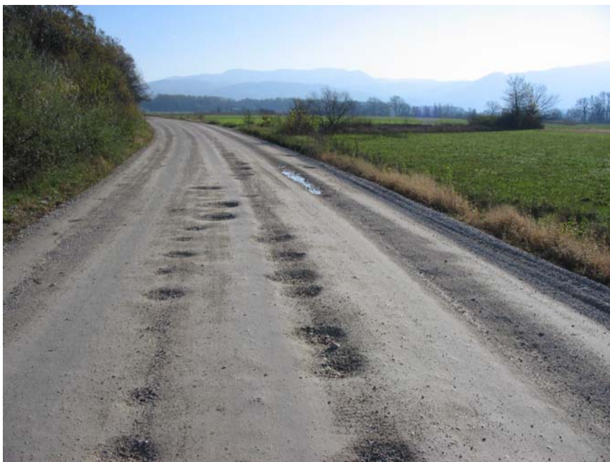
Example of potholes in the "ruts"
