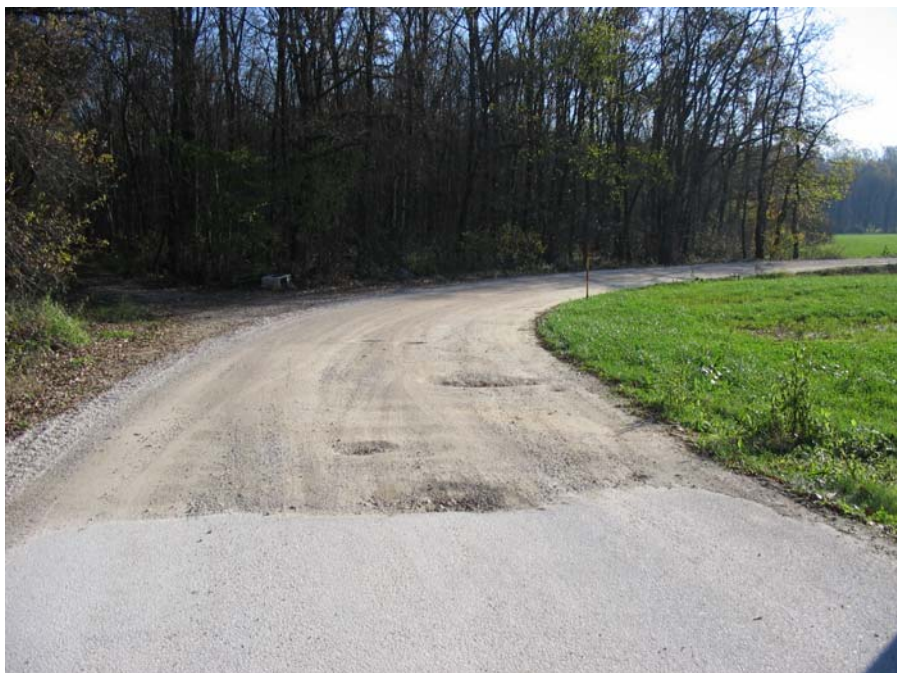
Example of individual potholes
