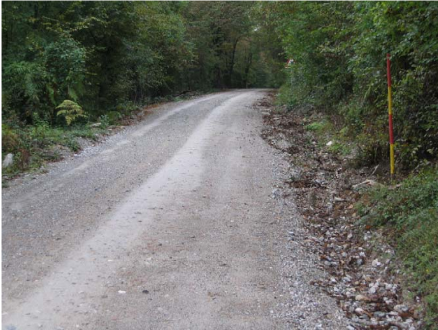
Example of consequences of water flowing along the right edge of the roadway
